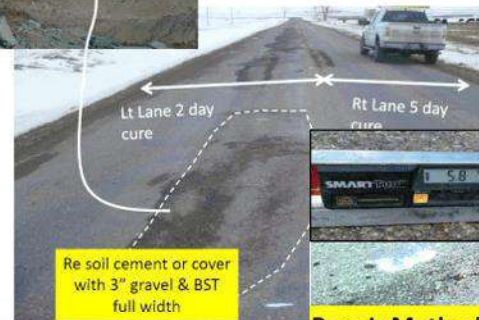
Damage by 200 Ton Oil Rig Movement (2011)
