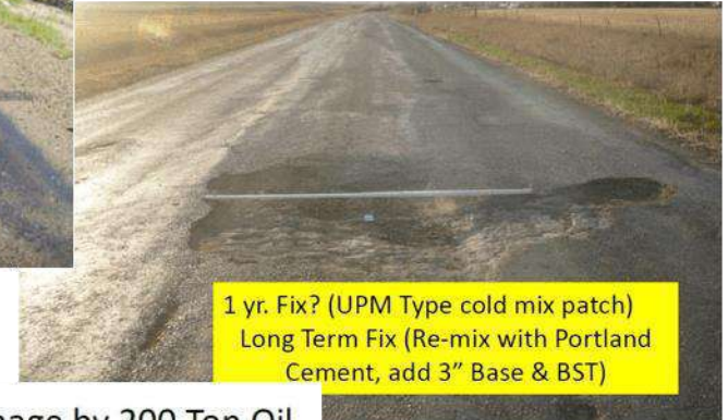
Damage by 200 Ton Oil Rig Movement (2011)
