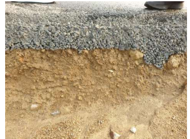
After 6 months Road Layer
